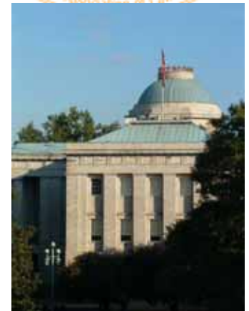
NC Capital Building
